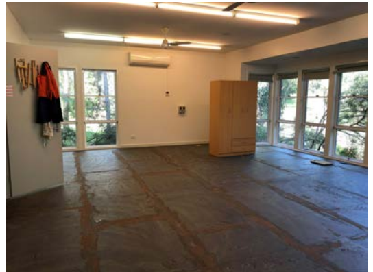
Preparing the floor in the art room for new vinyl
