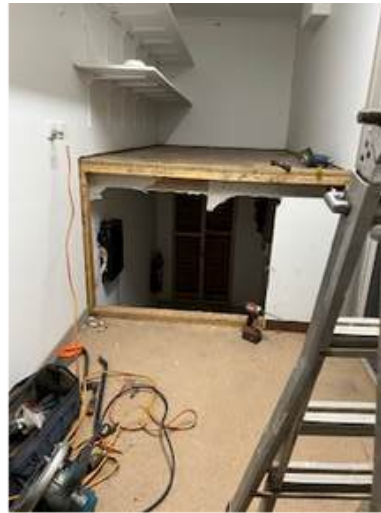
The internal access storage room - clearing out everything so construction on dropping the floor can be done
