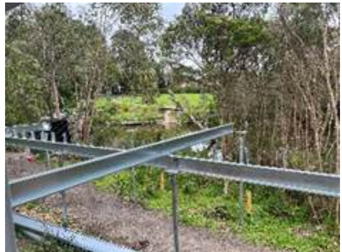
Laying the foundation posts and the steel framework
