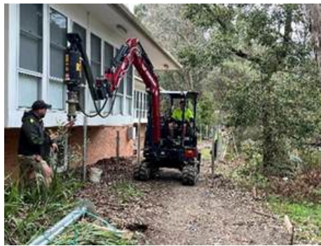
Laying the foundation posts and the steel framework
